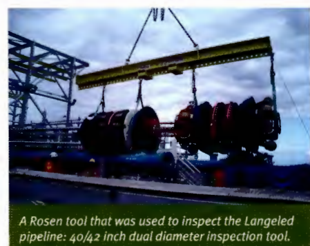
Launching the first MFL inspection tool.
