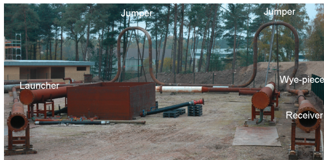
Figure 2: The 14"/18" test loop set up at the RTRC in Lingen, Germany, replicated all the important features and simulated the conditions of the pipeline to be inspected.
