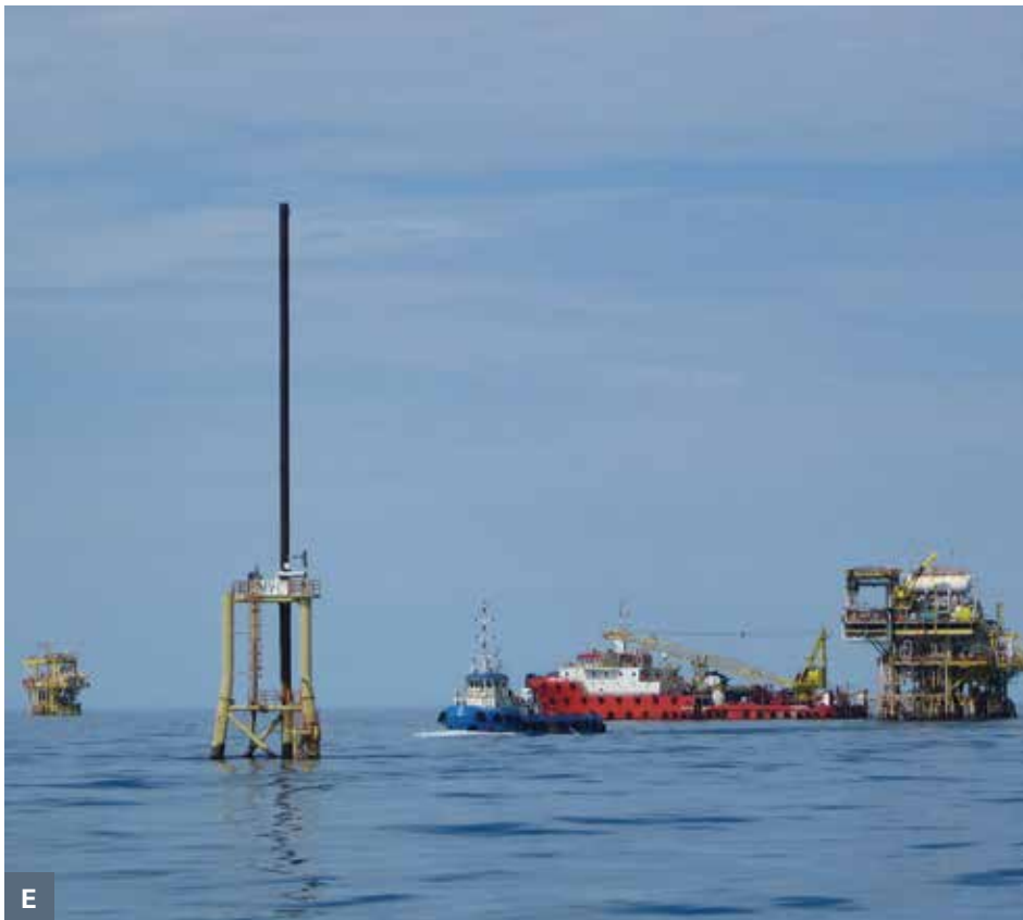
E: Vent lines reduce the risk of fire and explosion in processing systems by releasing the excessive gas at a safe distance from the platform.
