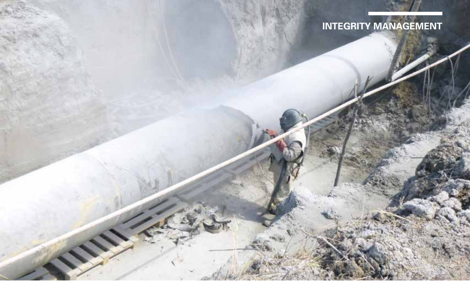
Repairs taking place as part of an integrity management plan.
