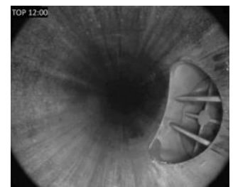
Figure 5: Hot tap with recessed pig bars
